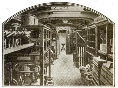
Inside one of the vans of the breakdown train, with tools and appliances arranged ready for instant use.
